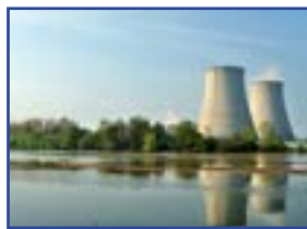
Nuclear access control
